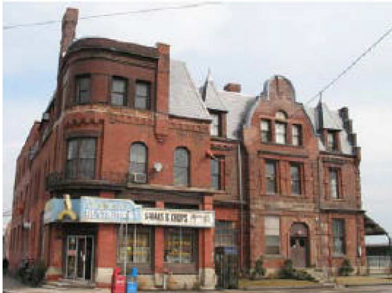
Canary Restaurant , Southeast Corner of Cherry St. and Front St. East (TRCA, 2004)
